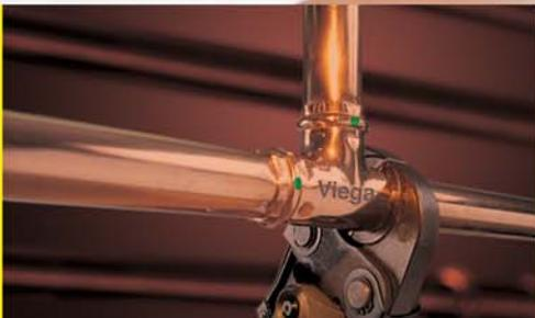
Viega ProPress fittings save you time and eliminate soldering or gluing for a safer, better air quality work environment.
